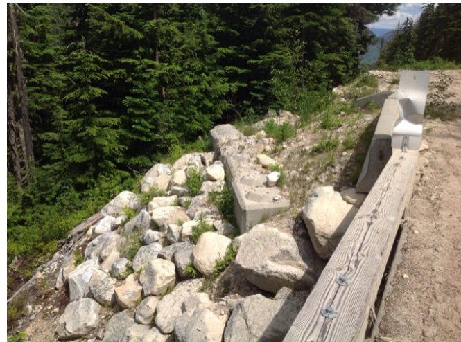
right bank wing wall
