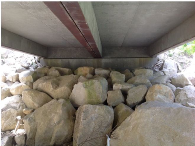
Left Bank Abutment when facing downstream
