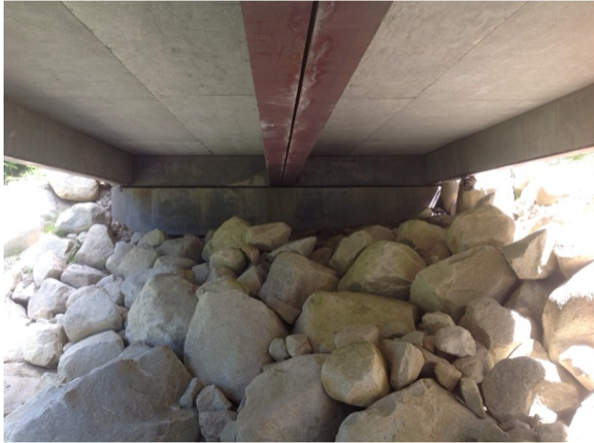
Right Bank Abutment when facing downstream
