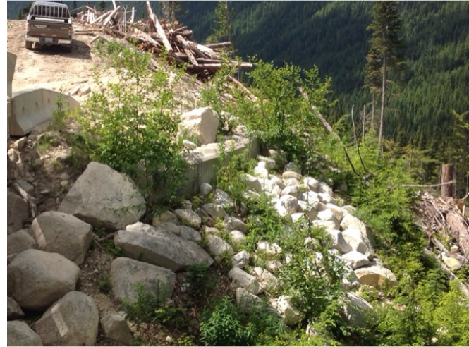
left bank wing wall
