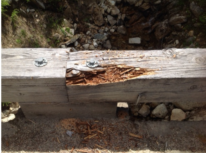
rotting guardrail
